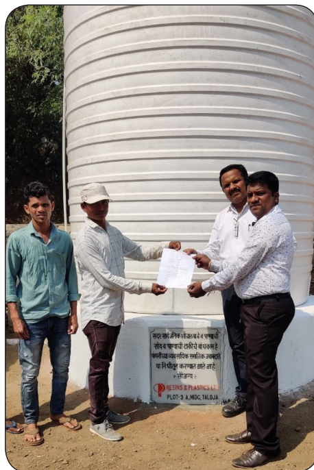
Supply of Water Storage Tank Civil Work - Village Kombal Tekdi, Panvel, Maharashtra
