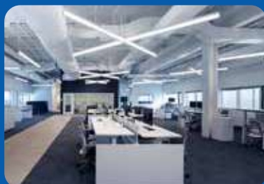
An adventure in lighting design starts now with an endless array of Philips ModiFly, which allows for ultimate flexibility in new age offices.
